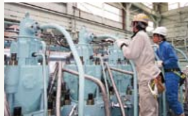
Shop test of critical equipment
