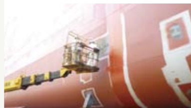
Welding inspection using an aerial work platform
